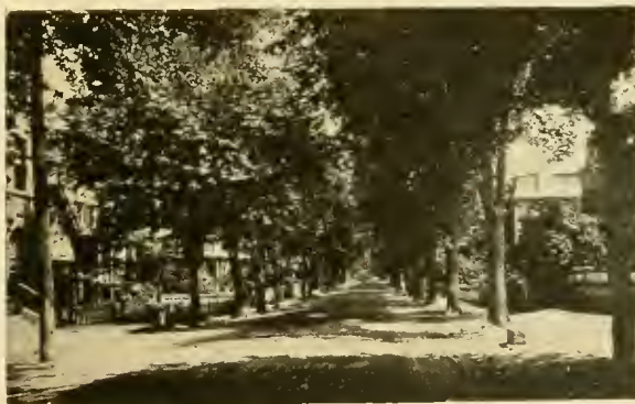
Washington Avenue and 173d Street, Before Widening
