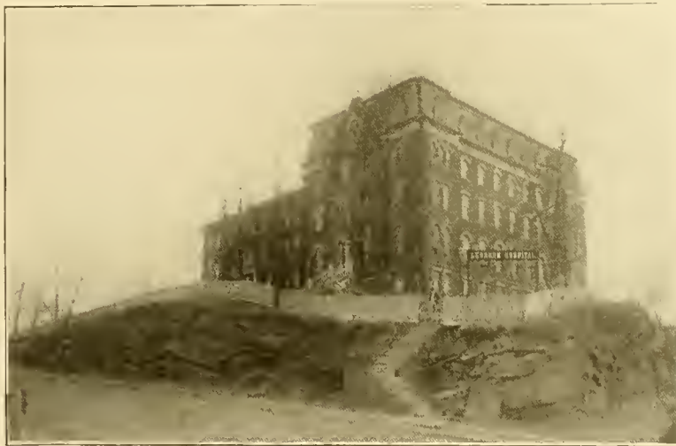
Lebanon Hospital, Westchester Avenue
