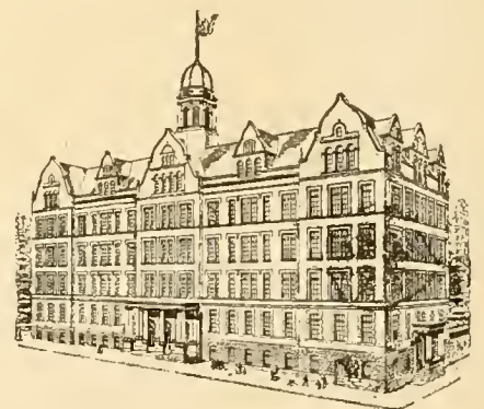
Public School No. 6, Locust Avenue, West Farms
