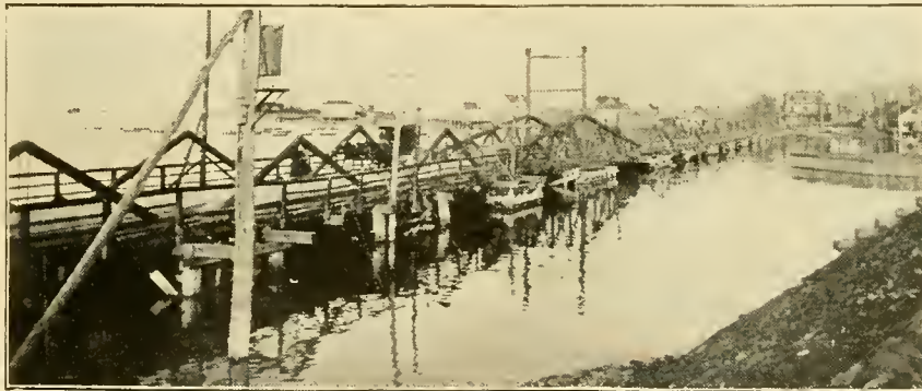
Old City Island Bridge
