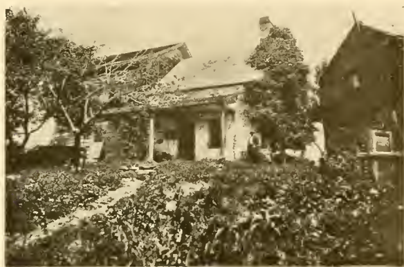
Old Hadley House, Moshulu
